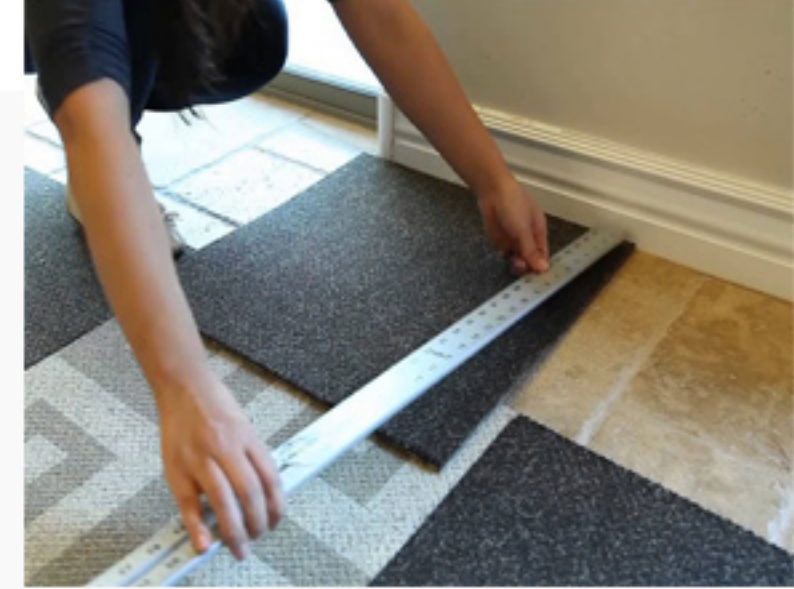
Carpet tile Installation
