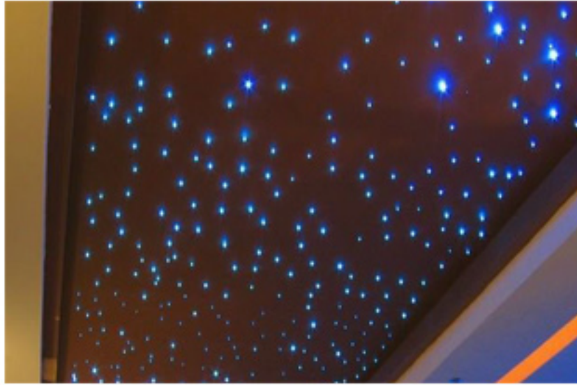
Fiber optic light installation
