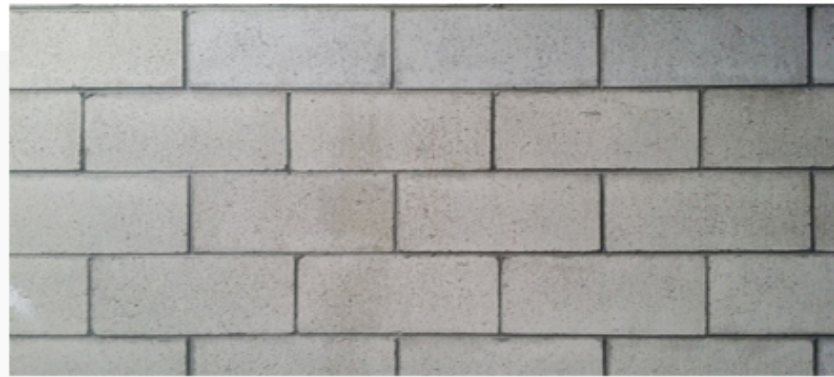
Block wall work
